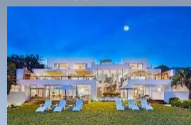
THE WHITE HOUSE BOUTIQUE VILLA
